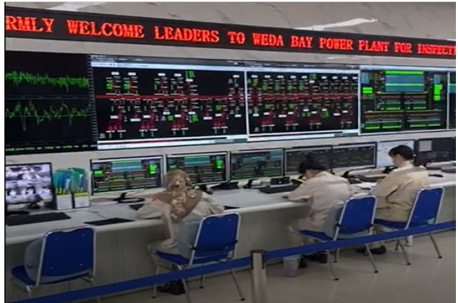
Weda Bay Power Plant control room
