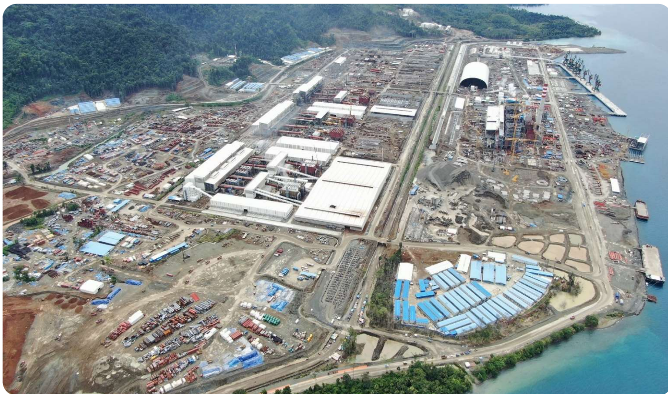
Aerial photo of the IWIP.
