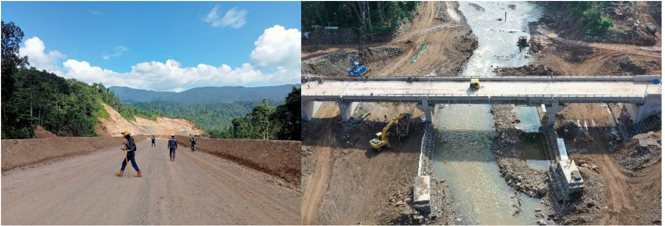
Mine haul road to bridge and bridge construction is nearing completion
