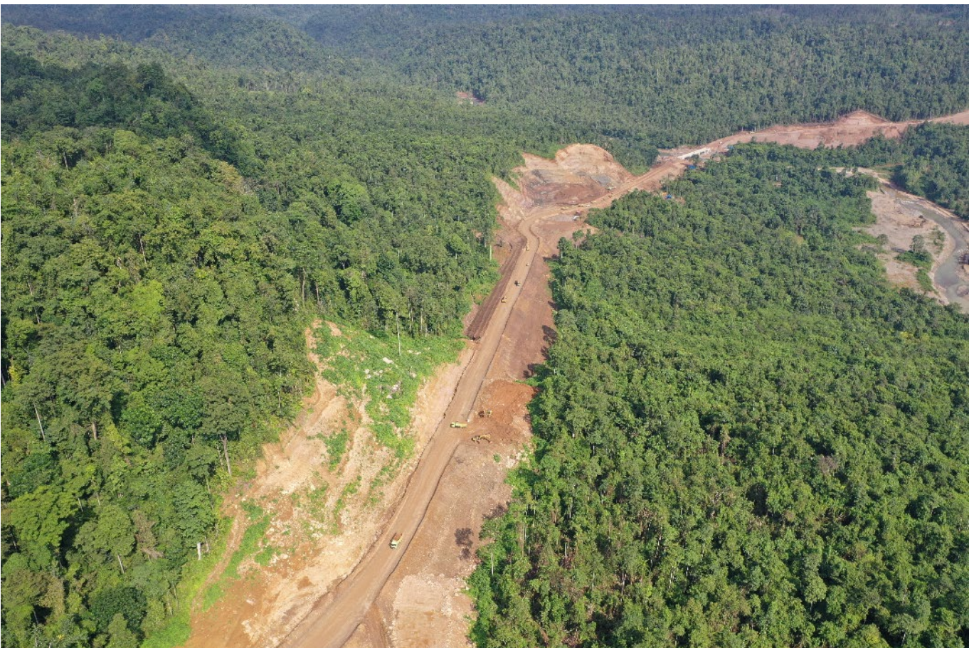
Haul road segment from IMIP river to IMIP is 98% complete
