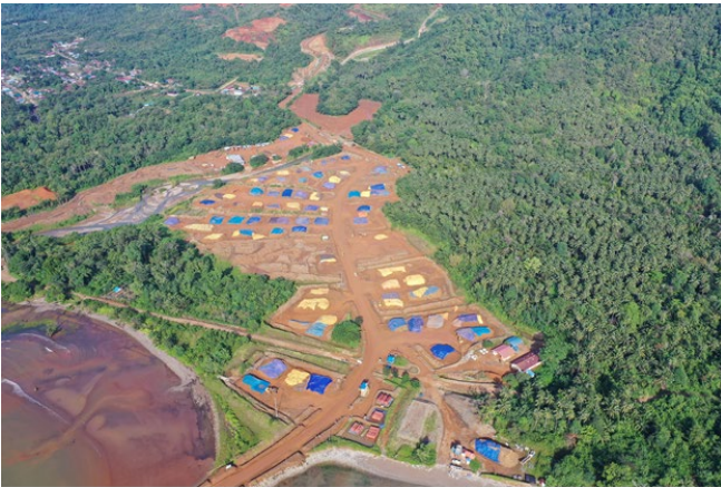
Stockpiles at Hengjaya Mine jetty
