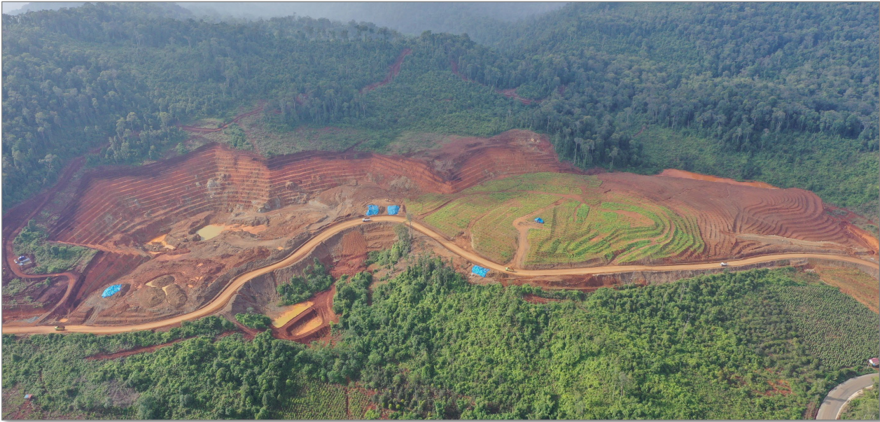
Central Pit rehabilitation has commenced
