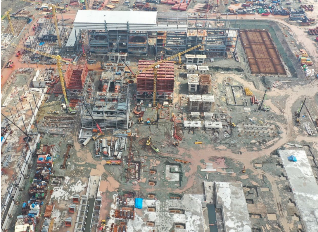
An aerial image of ONI construction progress within the IMIP
