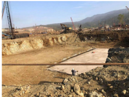
Foundations for Lines #3 and #4
