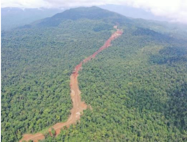
Main haul road works to IMIP
