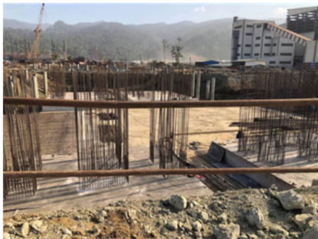
Foundations for Lines #1 and #2
