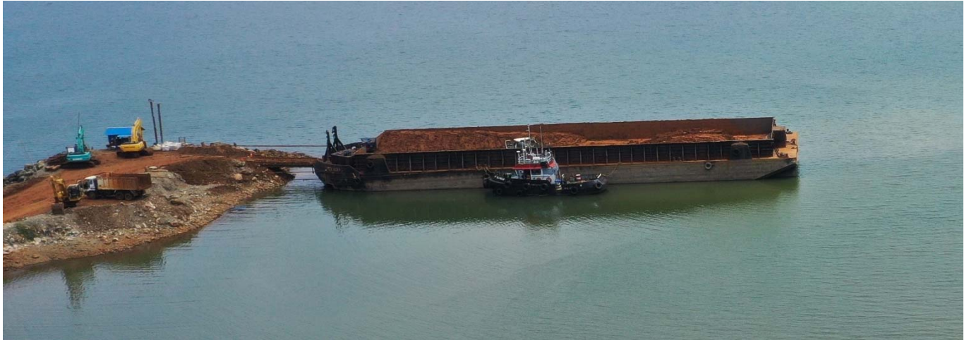
Aerial image of the Hengjaya Mine Jetty (to be upgraded) with 4,500 wmt barge moving to 7,500 wmt barge
