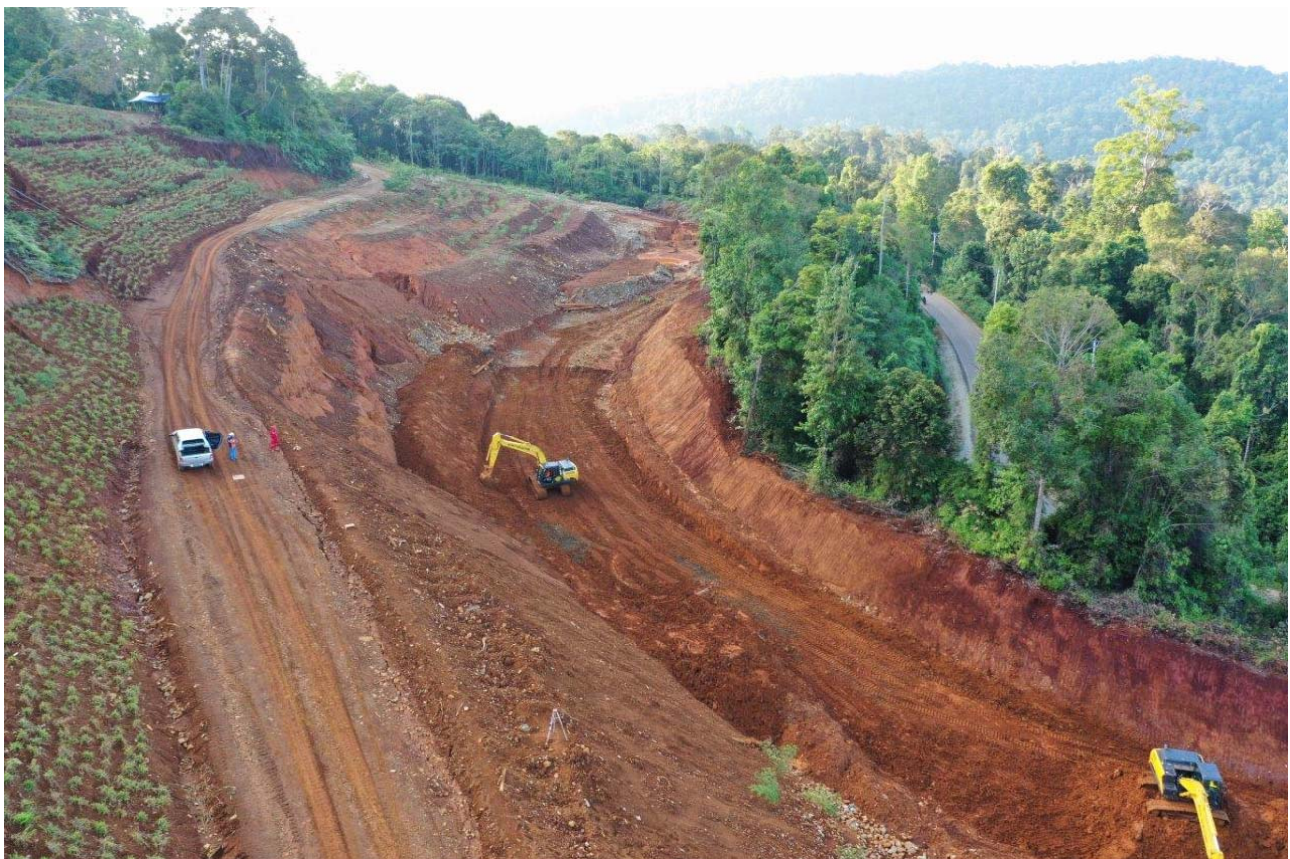
Aerial view of the haul road expansion
