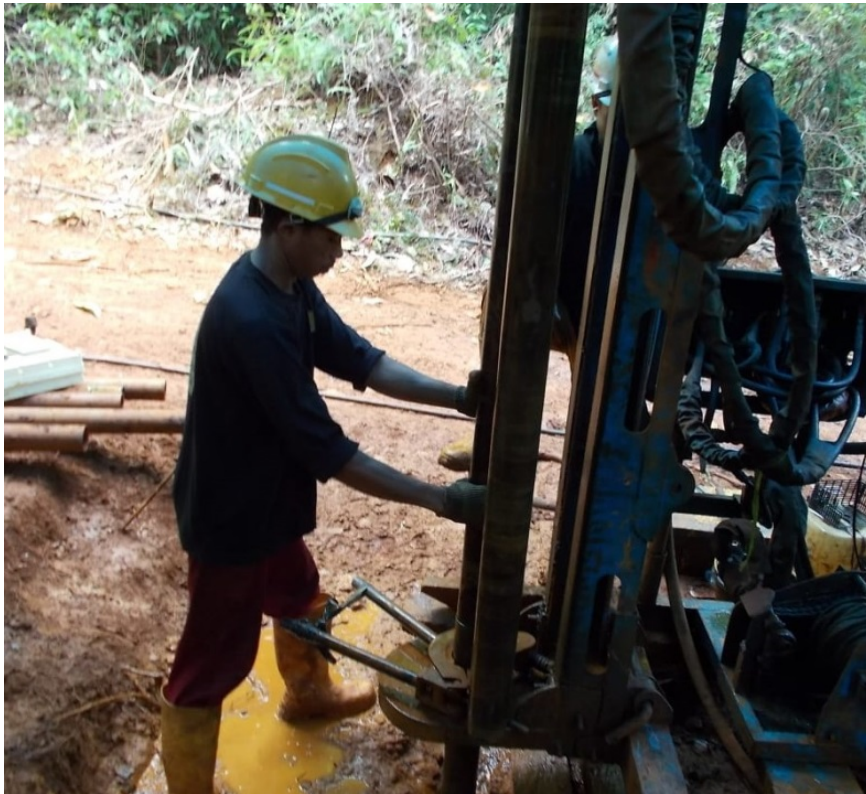
Completing drill rig set up at Bete Bete
