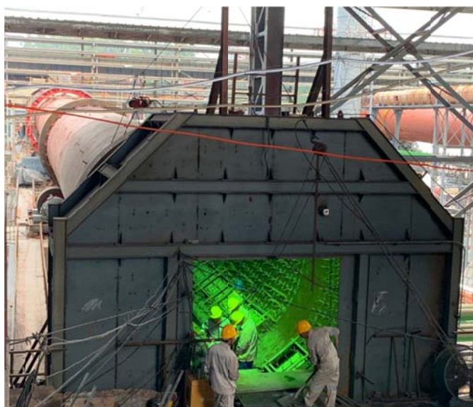
Lining of the Ranger Nickel rotary kilns with refractory brick
