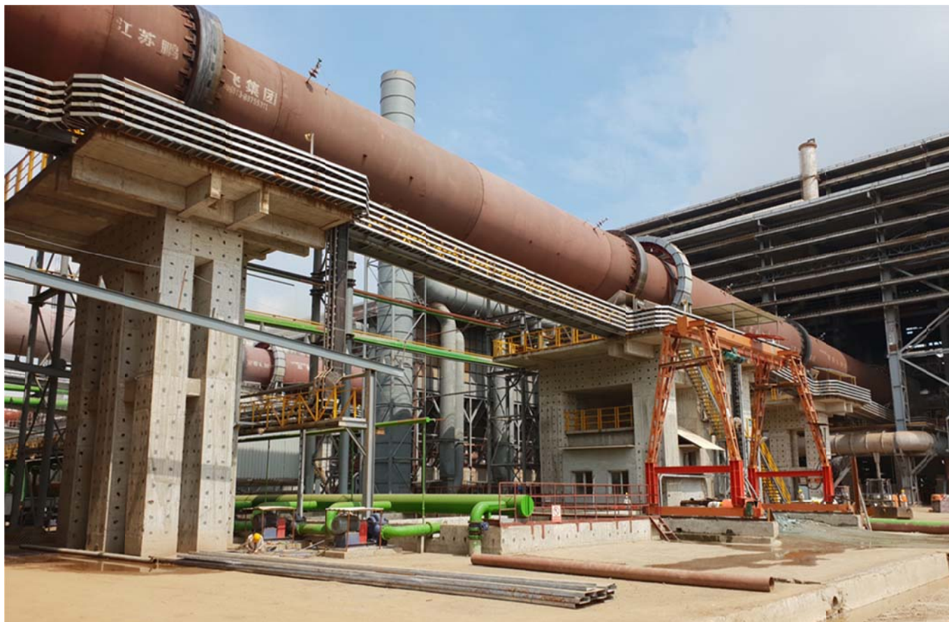
Construction progress at the Ranger Nickel Project
