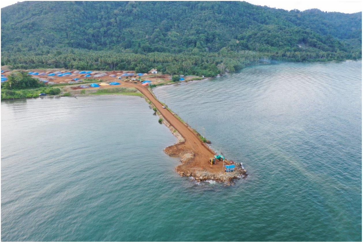
Aerial view of jetty currently undergoing expansion
