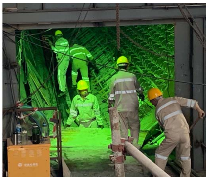
Lining of the Ranger Nickel rotary kilns with refractory brick
