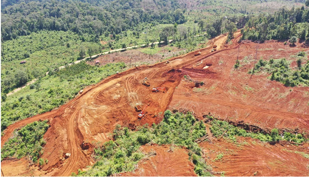
Central pit - Mining commenced in April 2020
