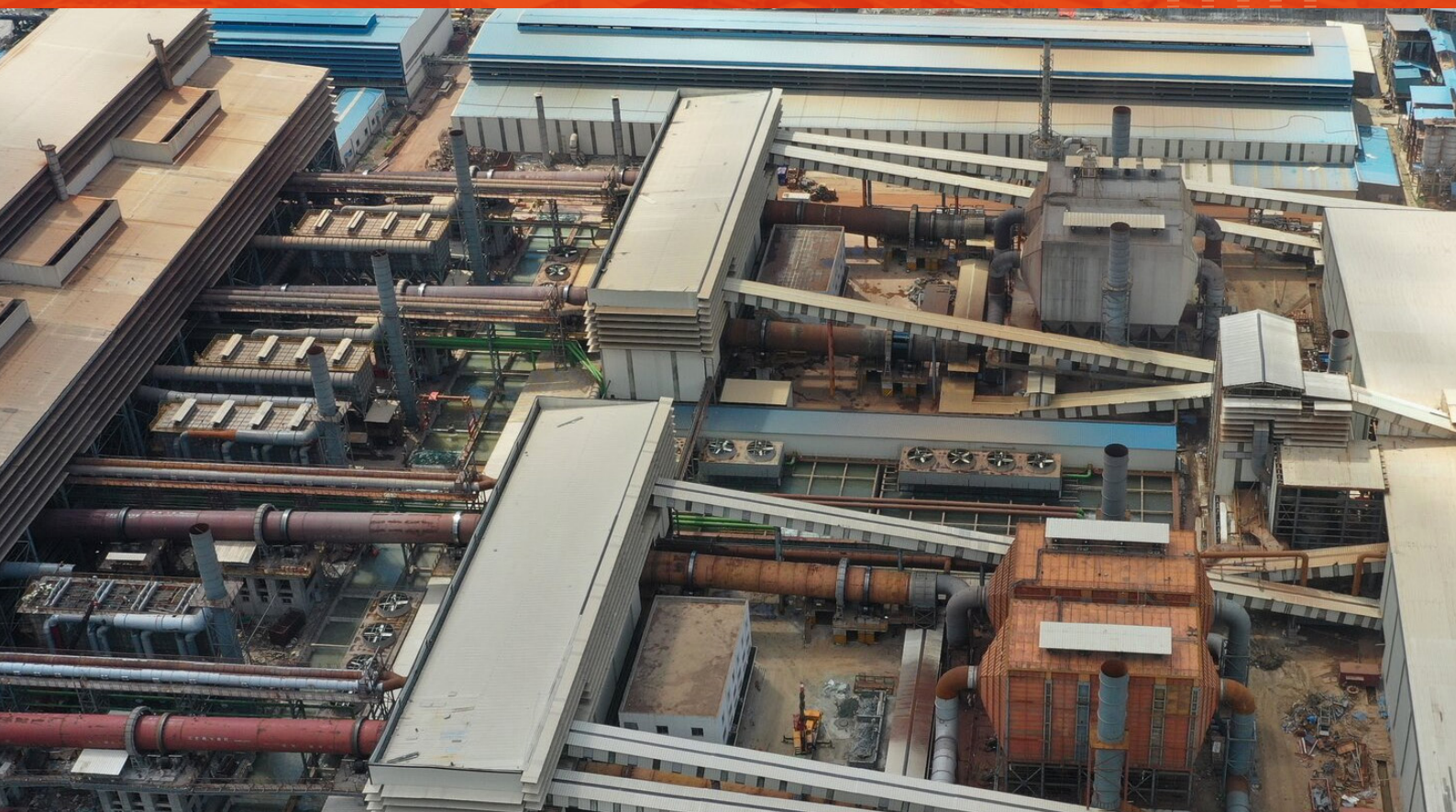
Aerial view showing Hengjaya Nickel and Ranger Nickel's RKEF lines
