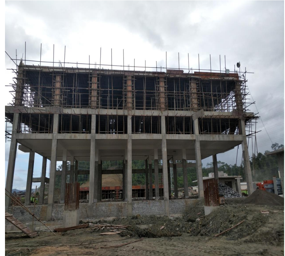
Electrical Switch Room
