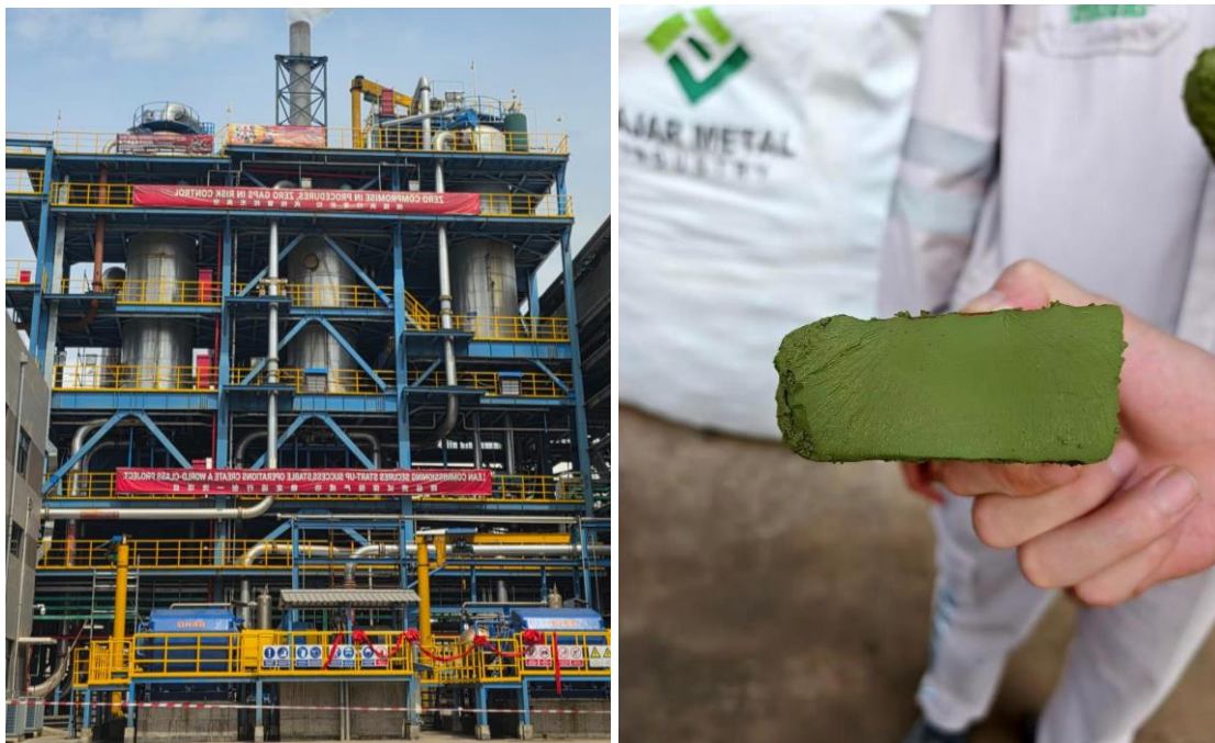
ENC plant and first MHP
