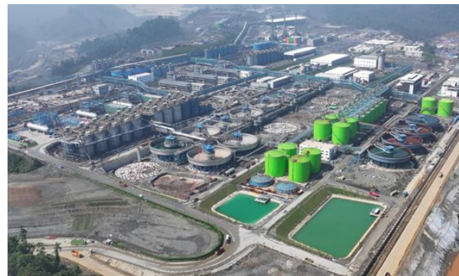
HPAL Smelter with integrated sulphuric acid and power plants
