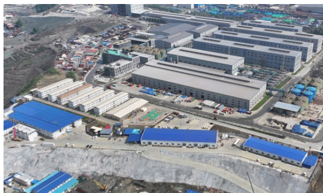
ENC integrated sulfate and cathode Refinery
