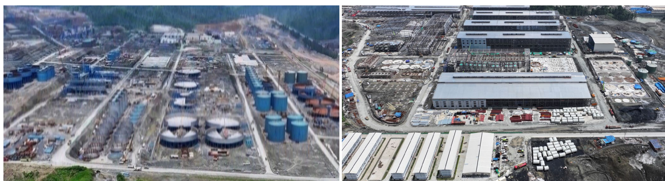
ENC HPAL (left) and sulfate and cathode refinery (right) construction progress
