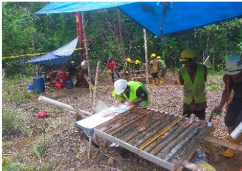
Photo 8 Logging cores at wellsite at IMM
