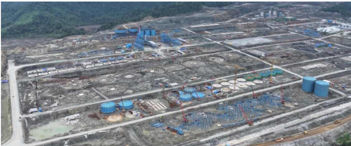
ENC HPAL construction progressing well
