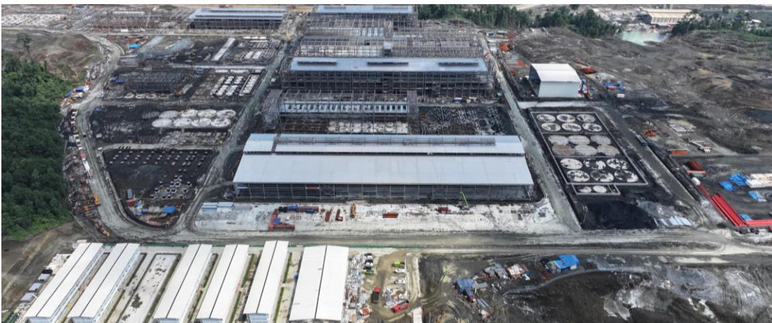
ENC sulphate and cathode refinery construction ahead of schedule
