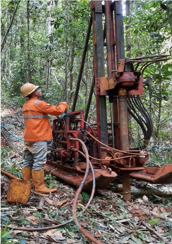
Photo 4 Dexdrill 200 operating at ETL
