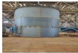
Acid plant drying tower
