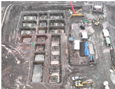
Sulfur storage yard and loading system
