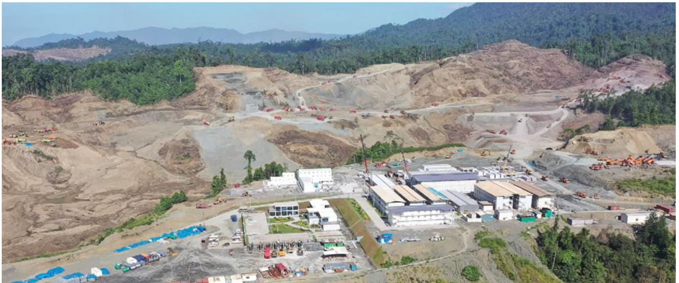
***Office and staff buildings completed with earthworks and footings at ENC largely complete in readiness for concrete pouring and plant erection***
